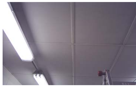
Vinyl grid covers for rusted, pitted or discolored grid.
