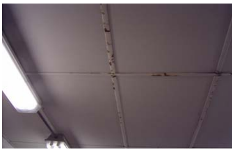
Vinyl grid covers for rusted, pitted or discolored grid.
